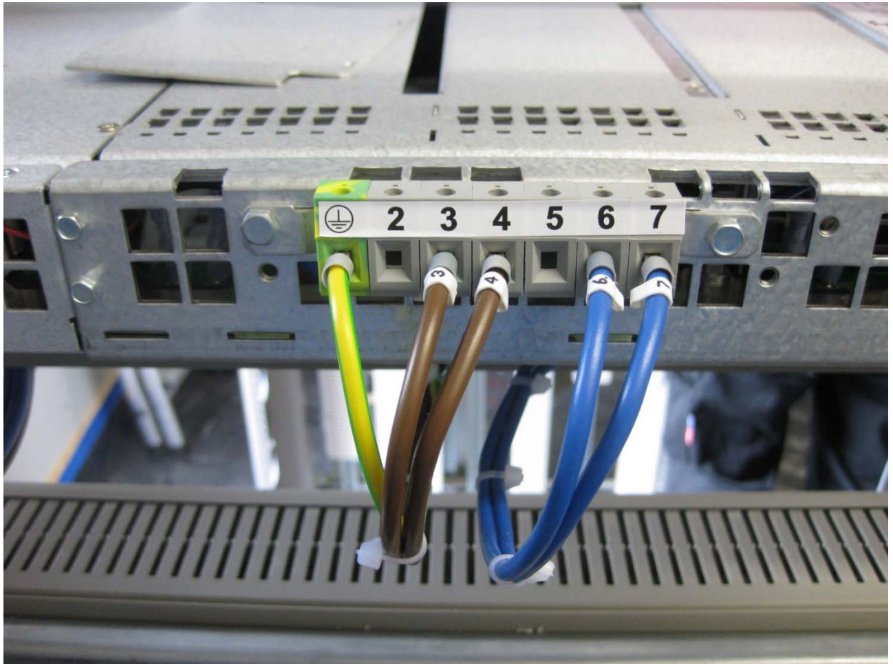
Figure 17. AC Power Wiring
