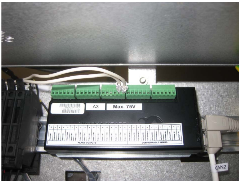
Figure 27. Alarm Wiring
